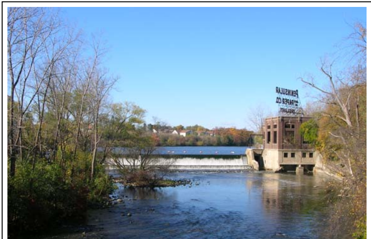
Figure 5-1: The 1867 Edison powerhouse , in Peninsular Park, is an Ypsilanti landmark. Seeking a private partner may be a way to both address the structure's physical deterioration and add a use to the park that can serve as a focal point for the neighborhood.
