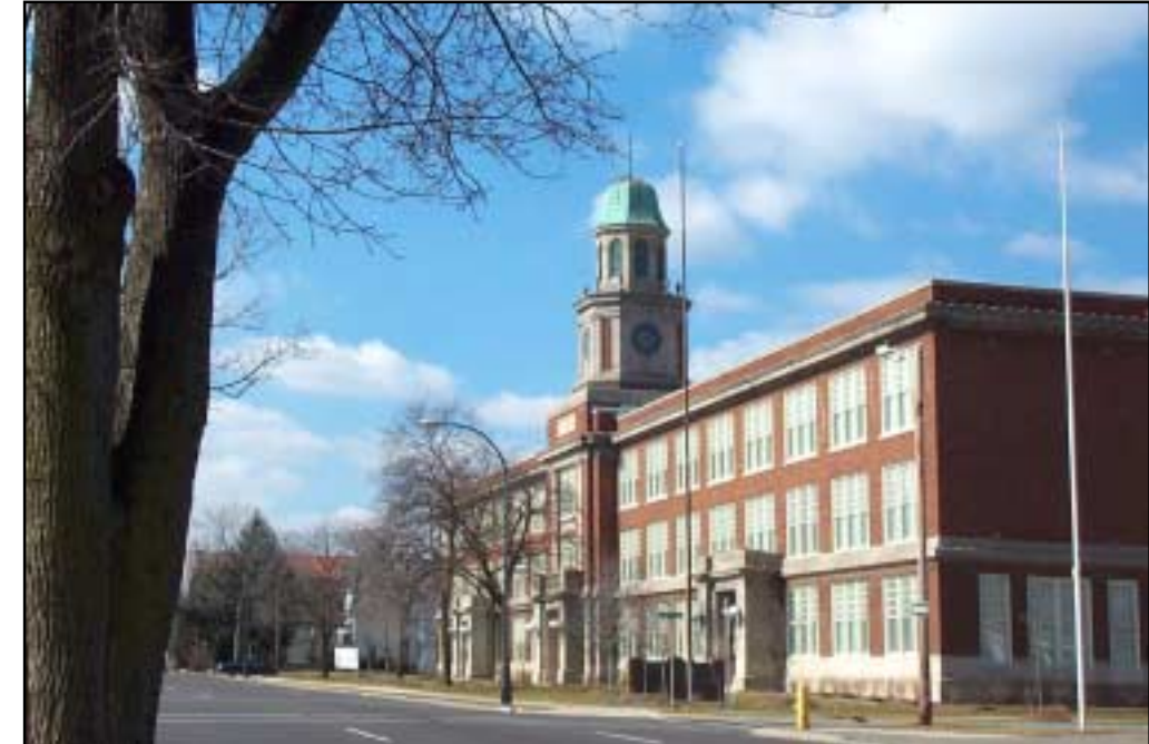
Above: The former Ypsilanti High School is now a successful senior housing development.
