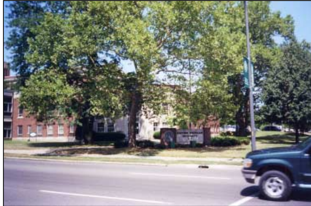
Above: Corner of Cross and Perrin: the location of the future parking deck.
